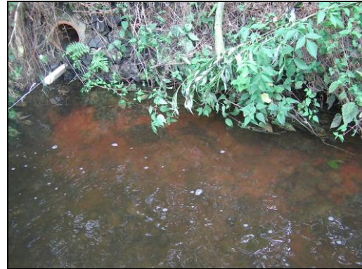
Fig. 12 Coarse sediment deposited on channel bed in the vicinity of the outfall
