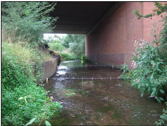
Fig. 1 Receiving Water Reach - looking upstream from mid-reach
